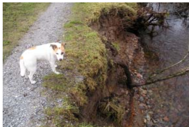
Bank Erosion at the Inverlocy River
